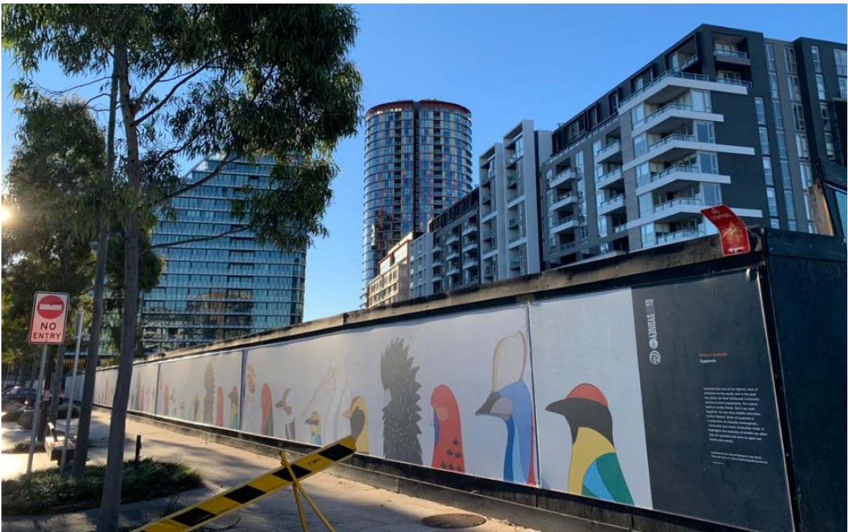
Figure 4: 'Stage 3' site viewed from the corner of Green Square Plaza and Paul Street, looking west
