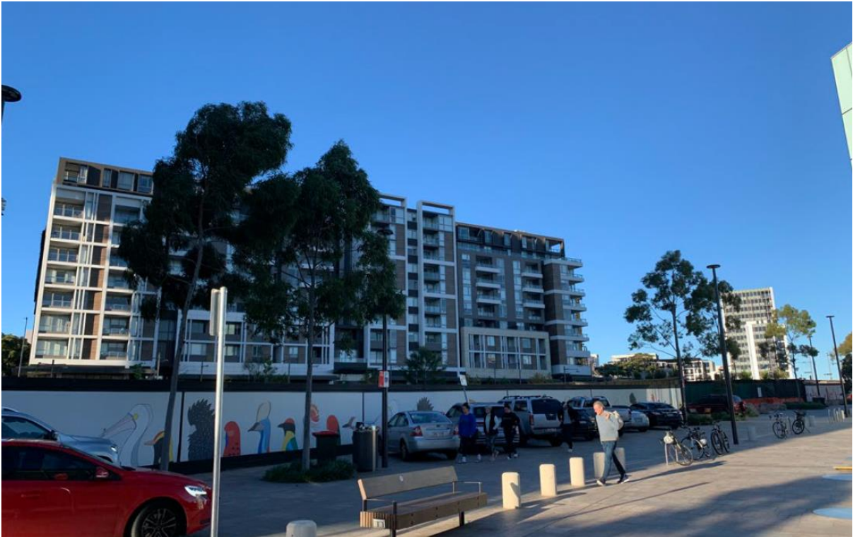
Figure 1: 'Stage 3' site viewed from Green Square Plaza, looking north-east
